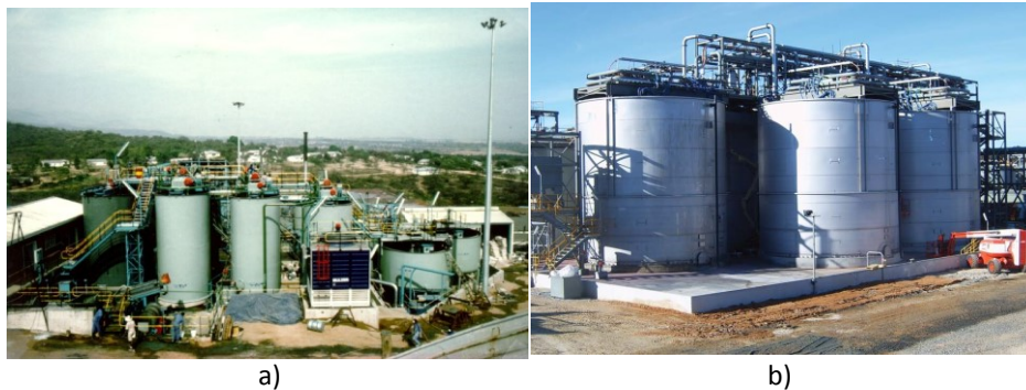
Figure 12 Bioleaching tanks of refractory gold in a) South Africa, b) Kazakhstan
